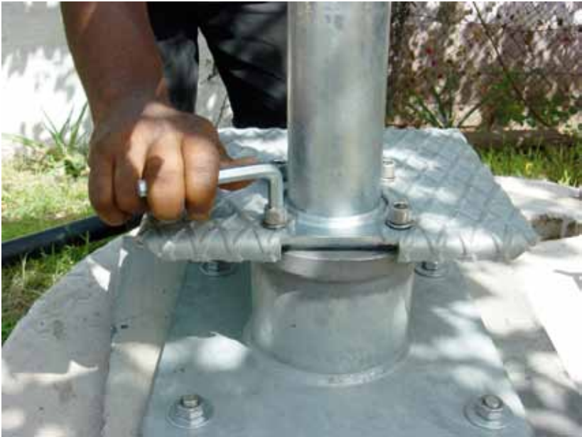
11. Tighten the all four bolts alternatively by using the allen key
