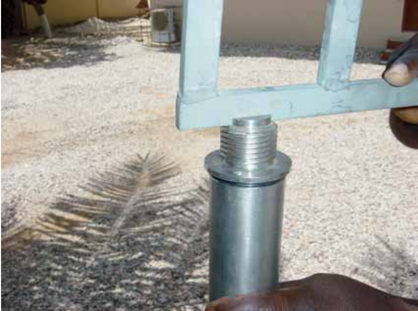
34. Fasten the handle nipple to the handle T-bar using the F-key.
